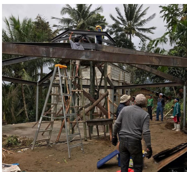
The steel made it to Lantawen
