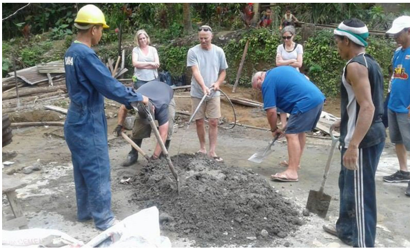
Three become one as the concrete is mixed
